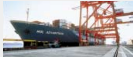
The new Ohi container terminal
