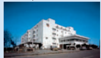
MOL Ohi Physical Distribution Center
