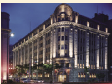
MOL (Kobe) building (when illumination is turned on)
