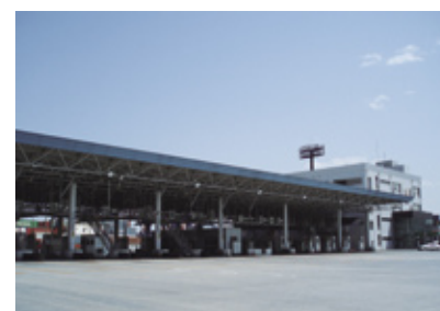
Gate 4 at International Container Terminal Co., Ltd. in Tokyo (TICT) Tokyo Bay Ohi Container Wharf
