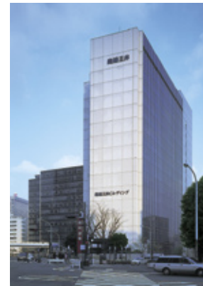
MOL Head Office Building
