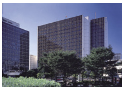
MOL Head Office Building
