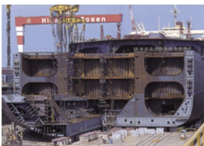
Double-hull structure
