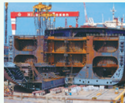
Double-hull structure
