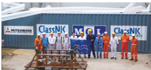
The installed packaged container ballast water treatment system
