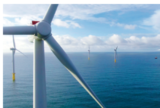
Offshore wind farm
