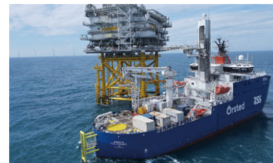
SOV transporting maintenance technicians to an offshore substation
