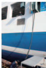
Onshore power supply system
