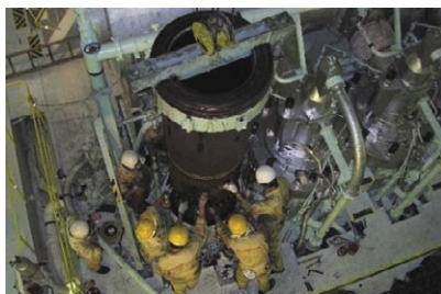
Engine Department: Removing a piston from the engine
