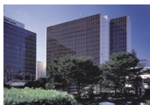
MOL Head Office Building
