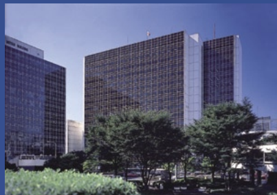
MOL Head Office Building
